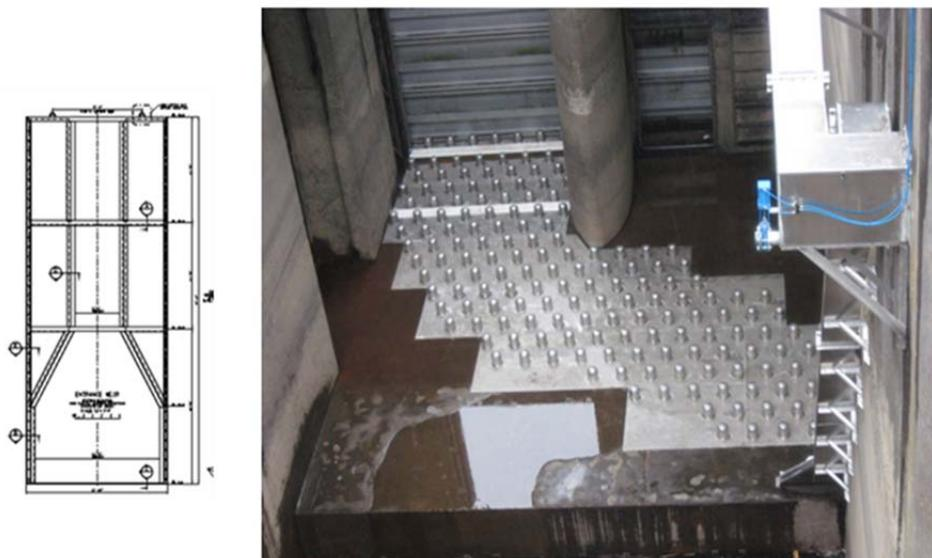
Figure 2. Variable-width entrance weir (line drawing, left) and Bonneville Dam Cascades Island entrance during installation of bollards, Lamprey Passage System (LPS, ascending wall to right in photo), and HD-PIT antennas (white bars spanning opening near entrance bulk head).
