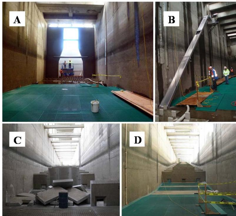
Figure 3. Modifications to the John Day Dam north fishway entrance area: A) variable-width entrance weir, bollard field, and closed entrance slot (new concrete on left wall); B) lamprey passage structure (with bollard field in foreground); C) removal of concrete weirs; and D) completed fishway with concrete weirs removed.
