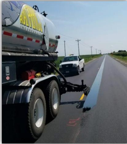
Placed by pressure distributor with mechanical agitation in tank
